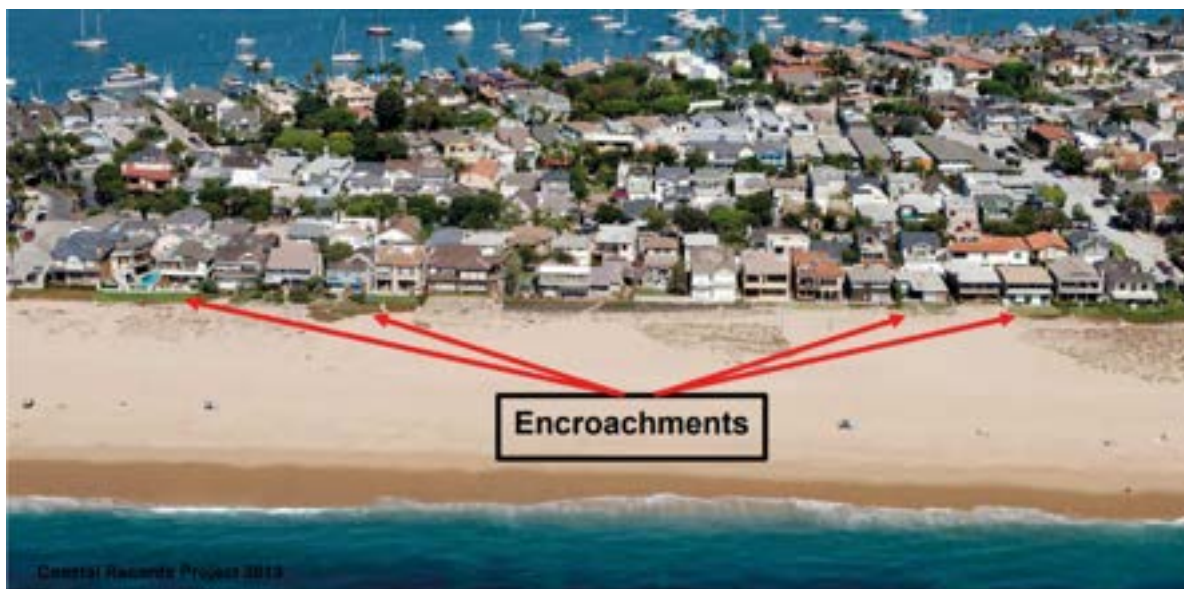
Figure N°14. Private residential encroachments on public beach, ordered to be removed, Newport, CA
